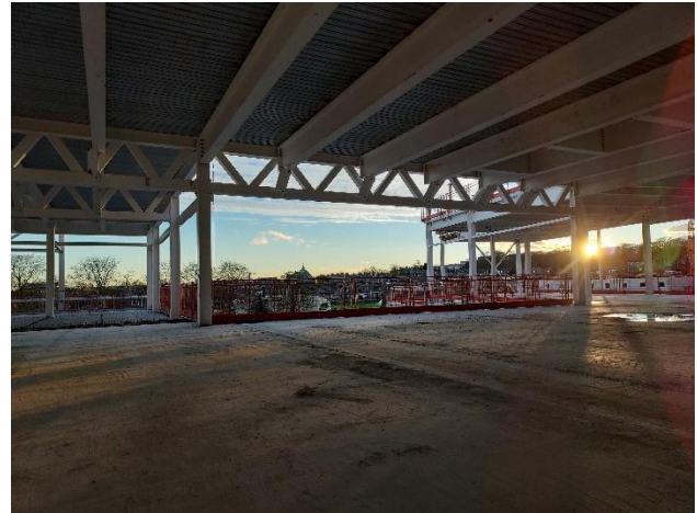
Image taken from the first floor of The ANCHOR Centre
