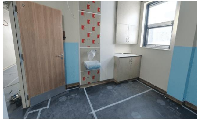
The ANCHOR Centre Ground Floor south – typical consulting room.
