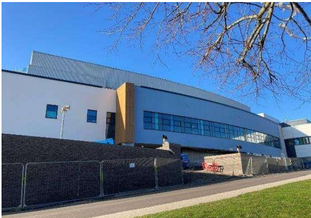
The ANCHOR Centre – east elevation (main entrance)
