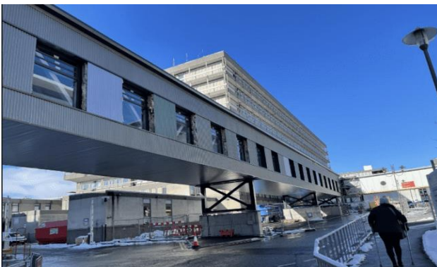
Baird north - new link bridge joining The Baird Family Hospital to Aberdeen Royal Infirmary (ARI) and Royal Aberdeen Children's Hospital (RACH).
