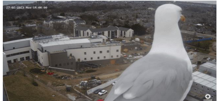
The ANCHOR Centre west elevation - A "bird's eye" view of
