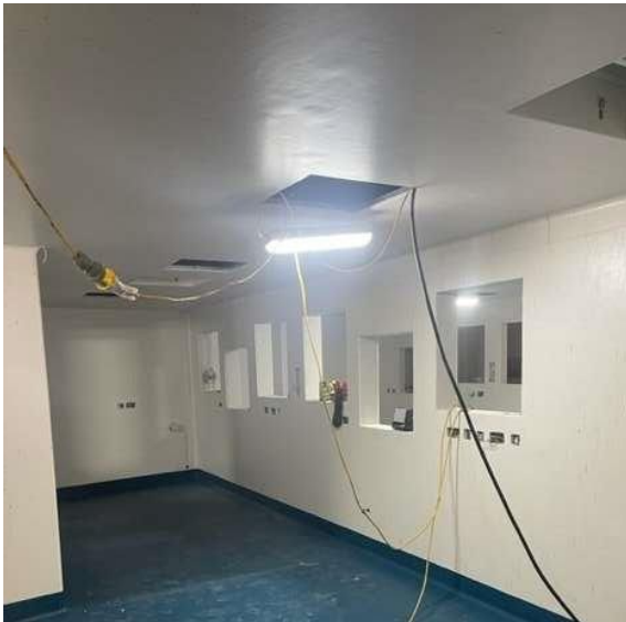
The ANCHOR Centre – Lower Ground Floor Aseptic Suite Outer Support Room
