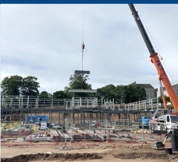
Mortuary progress looking South from Foresterhill Road:
