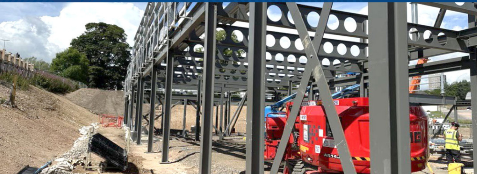
Zone 1 steelwork line and levelled.
